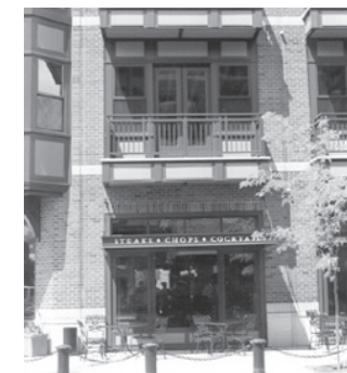
FIG. 4 - REINFORCE THE UNDERLYING STRUCTURE OF THE BUILDING. NOTICE HOW THE BRICK MASONRY PIERS AND SPANDELS DIVIDE THE BUILDING INTO INDIVIDUAL STOREFRONT BAYS AND UPPER-STORY FAÇADE OPENINGS.
