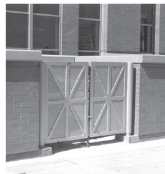
FIG. 12 - USE SOLID MASONRY ENCLOSURES TO SCREEN TRASH DUMPSTERS FROM PUBLIC VIEW. NOTICE ALSO THE DURABLE METAL GATES.
