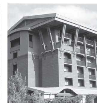
FIG. 2 - CROWN HOTEL BUILDINGS WITH A DISCERNABLE CAP DESIGNED TO TERMINATE THE TOP OF THE BUILDING. NOTICE HOW THE WIDELY OVERHANGING EAVE IS SUPPORTED BY AMPLE BRACKETS.
