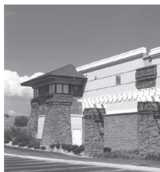
FIG. 11 - USE BUILDING MATERIALS TO ADD TEXTURE AND VISUAL INTEREST. NOTICE HOW THE RUGGED STONE BASE VISUALLY ANCHORS THE LARGE FORMAT BUILDING TO THE GROUND PLANE, WITH LIGHTER STUCCO WALLS OCCURRING ABOVE.
