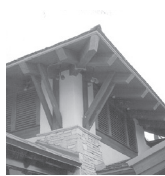
FIG. 9 - SUPPORT PITCHED ROOF OVERHANGS WITH BRACKETS OR CORBELS. NOTICE HOW THE AMPLE DIMENSIONAL TIMBER BRACKETS SUPPORT THE WIDELY OVERHANGING EAVE.
