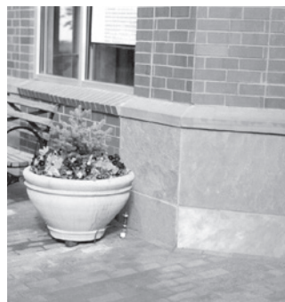
FIG. 11 - PROVIDE A DISTINGUISHABLE BASE OR BULKHEAD DESIGNED TO ANCHOR THE BUILDING TO THE GROUND PLANE. NOTICE HOW THE BUILDING BASE FUNCTIONS AS A PEDESTAL, VISUALLY SUPPORTING THE BUILDING MASS ABOVE.
