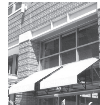
FIG. 5 - USE AWNINGS THAT CONFORM TO INDIVIDUAL STRUCTURAL BAYS WHILE ALLOWING LIGHT TO PENETRATE TRANSOM WINDOWS.
