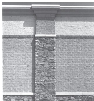
FIG. 9 - TERMINATE THE TOP OF LARGE FORMAT BUILDINGS WITH A ROOF CAP, SUCH AS A SUBSTANTIAL CORNICE ELEMENT THAT PROVIDES A BUILDING TERMINUOUS WHILE CREATING RICH SHADOW LINES. NOTICE ALSO THE AMPLE STONE PIER AND BUILDING BASE.
