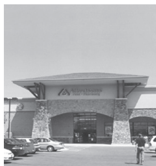
FIG. 12 - DEFINE LARGE FORMAT BUILDING ENTRANCES. NOTICE THE ENTRANCE PAVILLION COMPOSED OF SUBSTANTIAL STONE PIERS, DIMENSIONAL TIMBER BRACKETS, AND A DOMINANT ROOF CAP THAT "ANNOUNCES" ENTRANCE INTO THE STRUCTURE.
