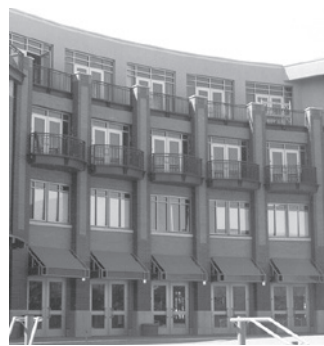
FIG. 7 - USE REPETITIVE WINDOW RHYTHMS TO DISTINGUISH UPPER STORY FAÇADES. NOTICE HOW THE BUILDING'S STRUCTURAL BAYS DEFINE INDIVIDUAL RECESSED WINDOW OPENINGS.
