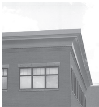
FIG. 8 - FOR FLAT ROOFS, TERMINATE THE TOP OF BUILDINGS WITH A DISTINCTIBLE ROOF CAP. NOTICE HOW THE SUBSTANTIAL PROTRUDING CORNICE ELEMENT TERMINATES THE TOP OF THE BUILDING.
