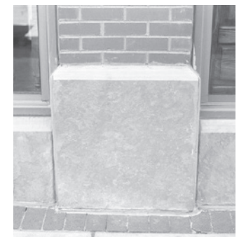
FIG. 6 - ANCHOR IN-LINE RETAIL STORE FRONTS TO THE GROUND PLANE. NOTICE HOW THE STONE VENEER BULKHEAD PROVIDES A SUBSTANTIAL BASE OR PEDISTAL FOR THE BUILDING TO REST UPON.
