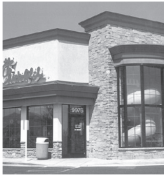
FIG. 7 - DESIGN PAD BUILDINGS, SUCH AS THIS FAST FOOD ESTABLISHMENT, TO REFLECT THE ARCHITECTURAL STYLE OF THE ENTIRE LIFESTYLE CENTER. NOTICE ALSO HOW THE CHILDREN'S PLAY STRUCTURES ARE LOCATED INTERNALLY WITHIN THE BUILDING.
